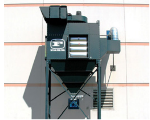
This heavy duty dust collector with explosion vent is designed to survive a combustible dust explosion with minimal damage.
